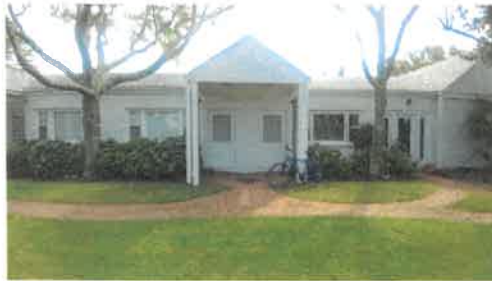
NORTH END OF BUILDING
